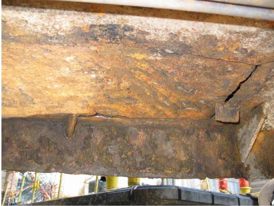
Figure 2-13. Example of cracking in web plates
