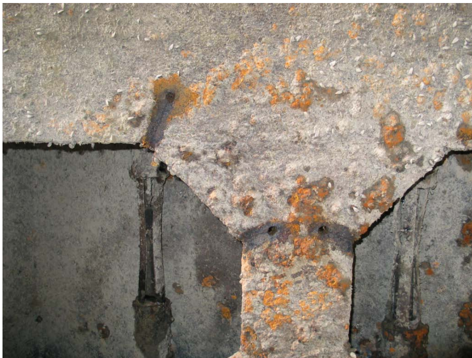
Figure 2-18. Example of drilling out crack tips to control fatigue cracking
