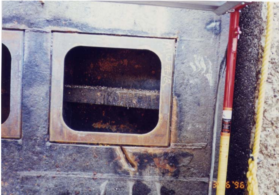
Figure 2-6. Example of window frame repair technique
