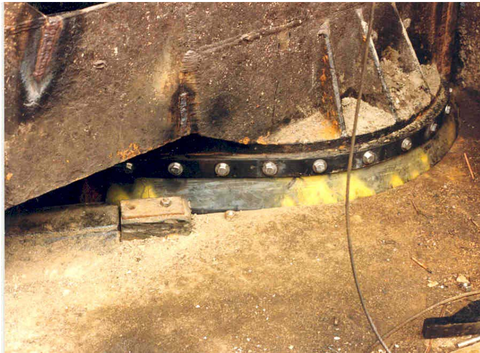
Figure 2-12. Example of cracking in the pintle connection
