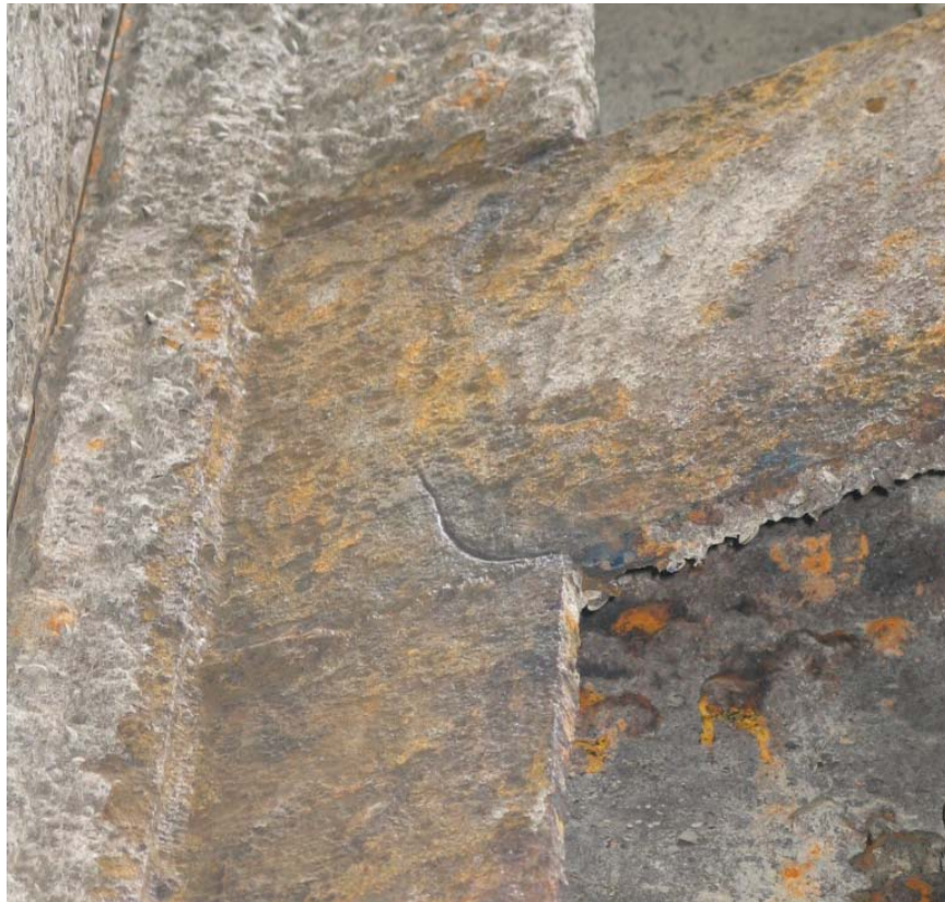
Figure 2-2. Example of fatigue crack at welded joint extending into horizontal girder flange
