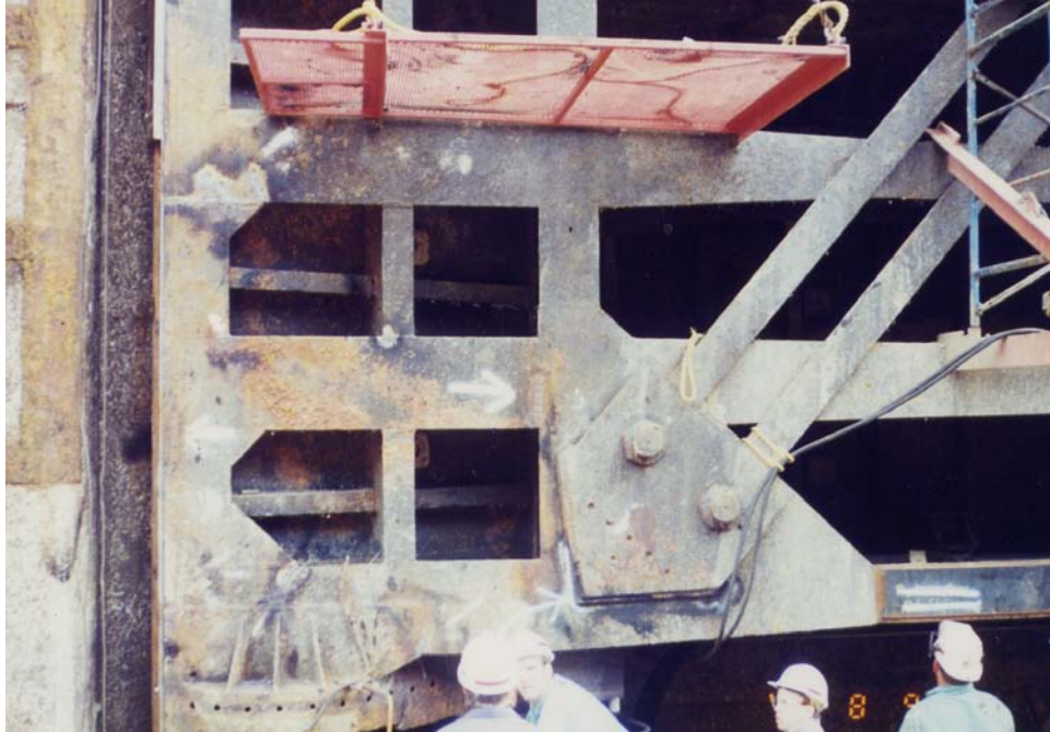
Figure 2-11. Example of cracking at the diagonal anchorage and pintle connection
