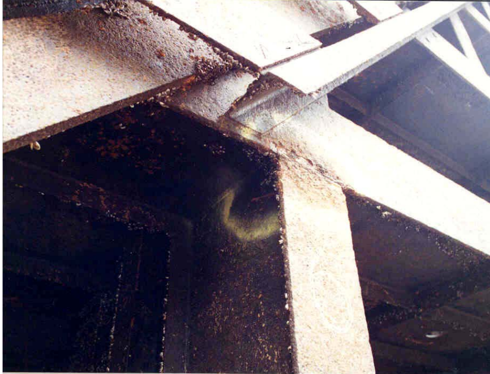
Figure 2-7. Cracking in girder flange connection near midspan with tension loads
