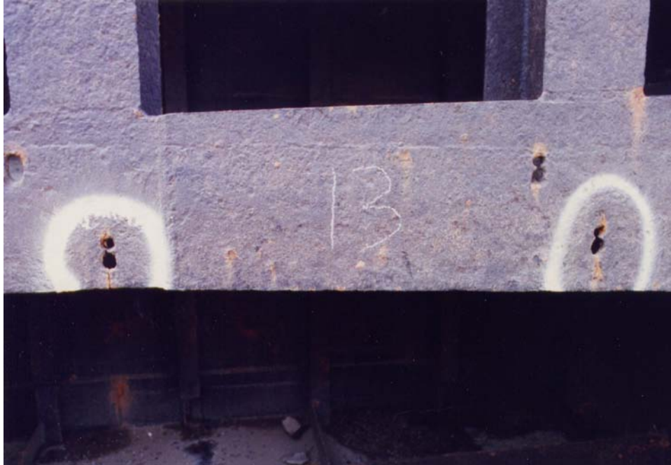
Figure 2-15. Example of miscellaneous cracking in girder flange
