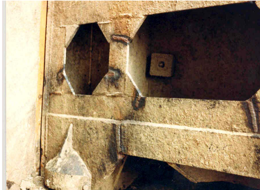
Figure 2-9. Cracking in girder and diaphragm flanges near quoin
