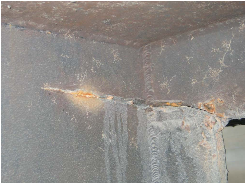
Figure 2-14. Example of crack in girder flange propagating into diaphragm web
