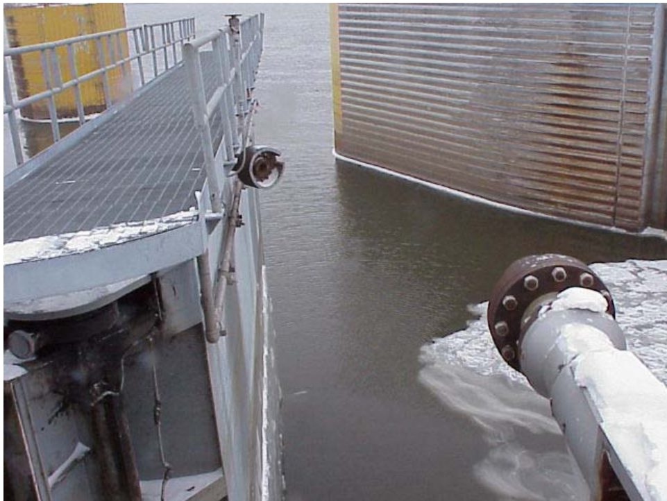
Figure 2-8. Example of fractured strut arm and anchor arm
