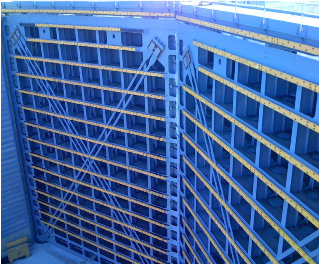
Figure 1-1. Horizontally framed miter gates in lock chamber, downstream view
