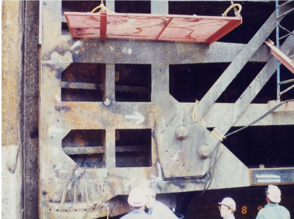
Figure C-1. Fatigue cracking in girder flange at diagonal anchor plate in Markland miter gates
