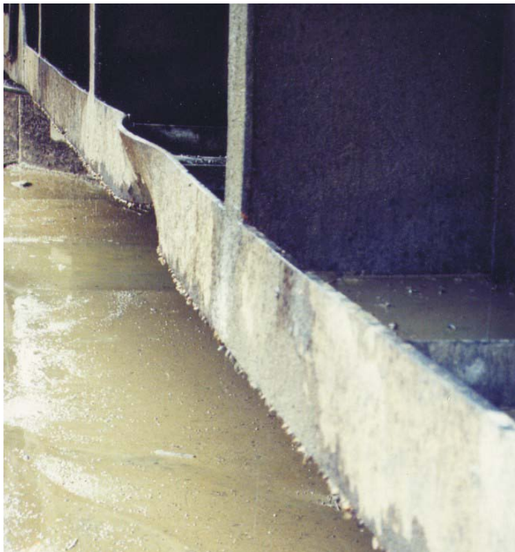
Figure 2-16. Example of damage from sill obstruction
