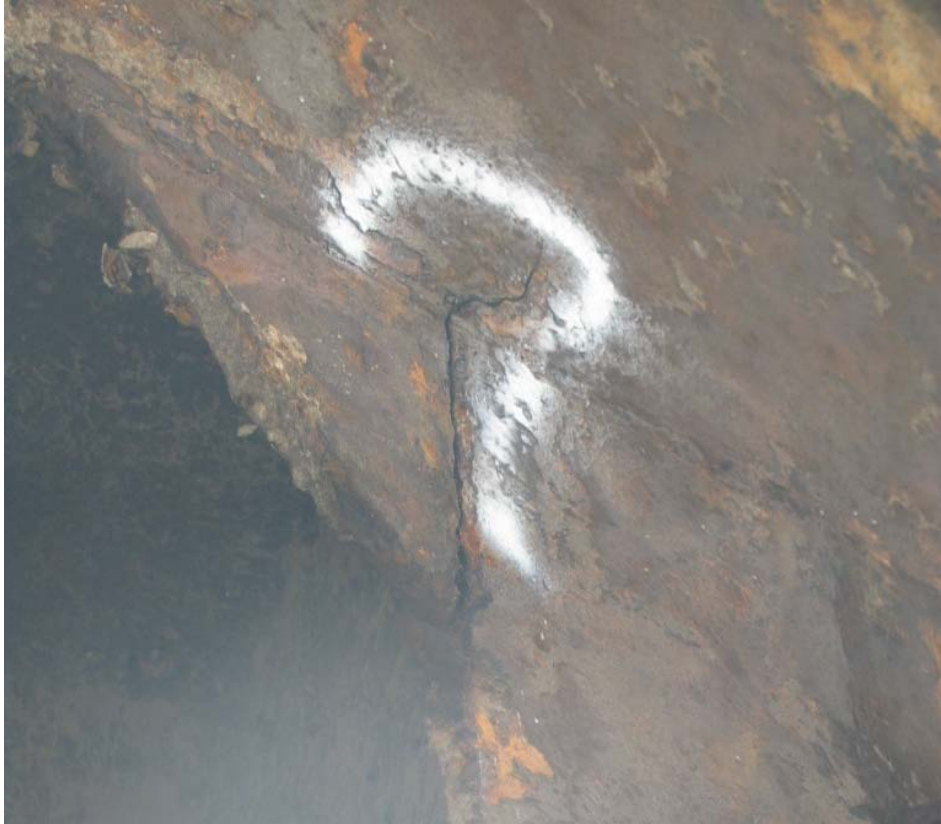
Figure 2-17. New cracking after gouging and rewelding a crack and adding gusset plate
