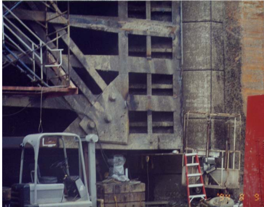
Figure 2-1. Fatigue cracking at welded joints of horizontal girders loaded in compression
